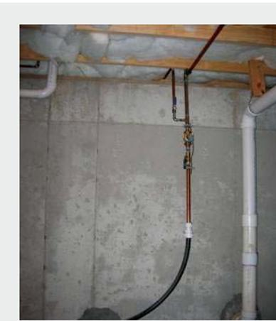
**E.** Polyethylene water service pipe entering the home through the concrete basement wall shown. White plastic adapter shown between polyethylene water service pipe and 3/4 inch copper water line. A short distance above the adapter is a pressure-reducing valve. To the right of water line is the 4-inch PVC pipe waste water line.
