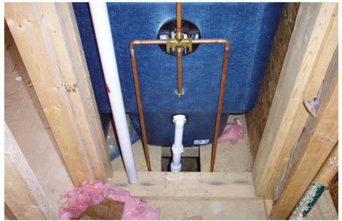
**D.** Mixing and antiscald water flow control, vent for fixture, hot and cold water lines, and bathtub overflow shown. At this point in construction, insulation might be considered for the hot water lines. Water service and waste water line.
