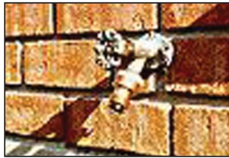
Figure 9.17. Hose Bib With Vacuum Breaker
